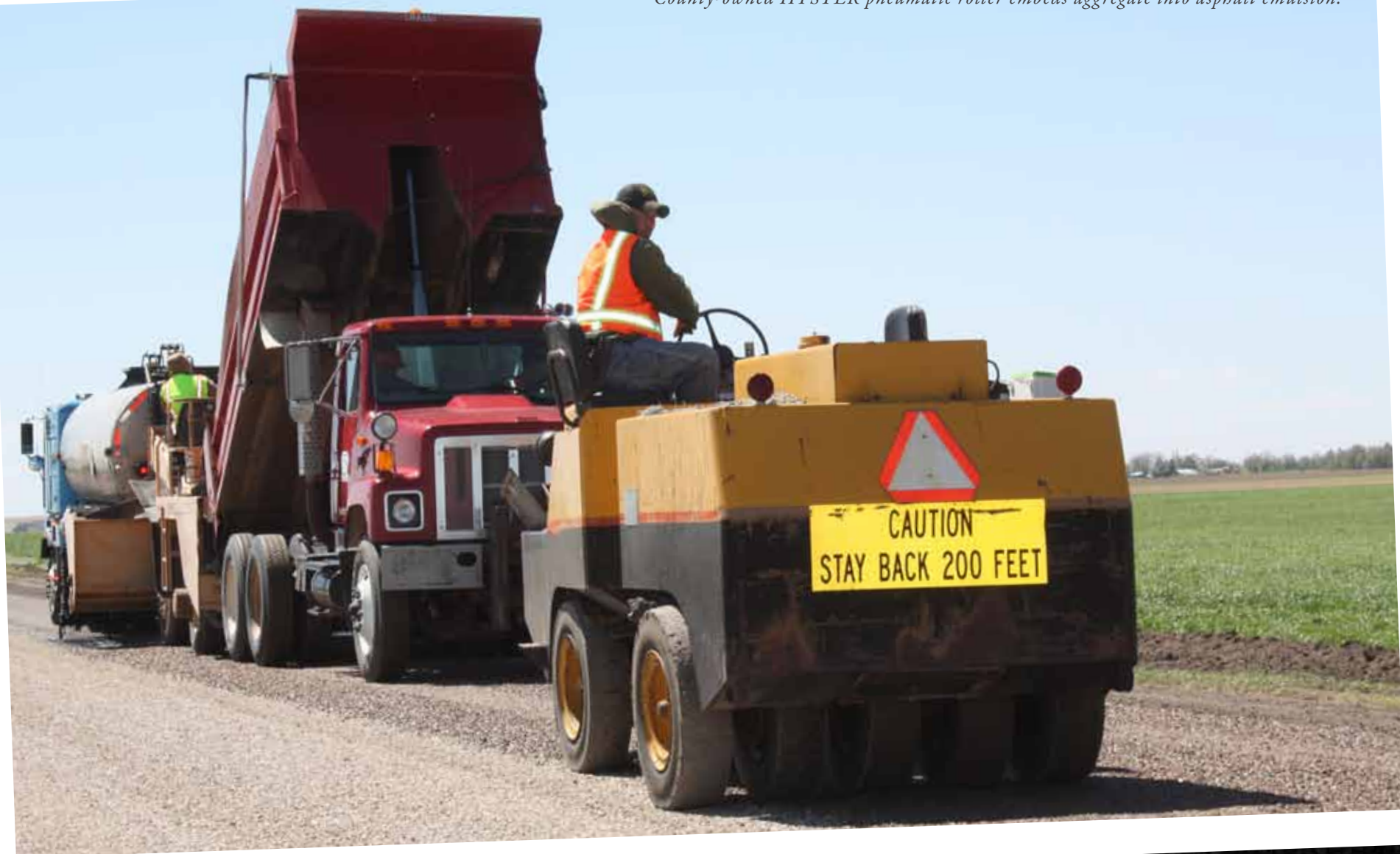
County-owned Hyster pneumatic roller embeds aggregate into asphalt emulsion.
