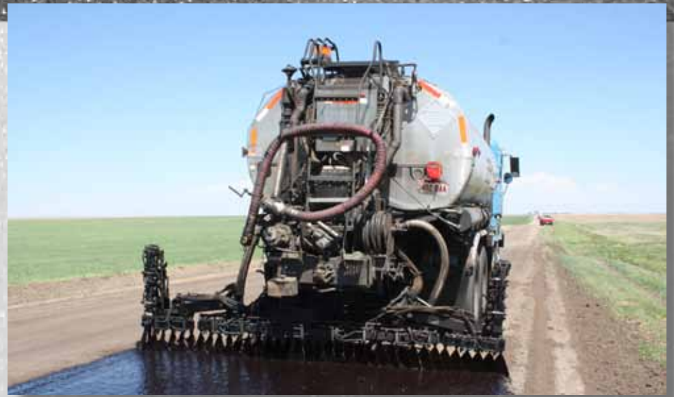
A BearCat distributor on a Freightliner chassis sprays COBITCO's CRS-2R emulsion modified with BASF SBR latex polymer at 0.65 gallons per square yard
